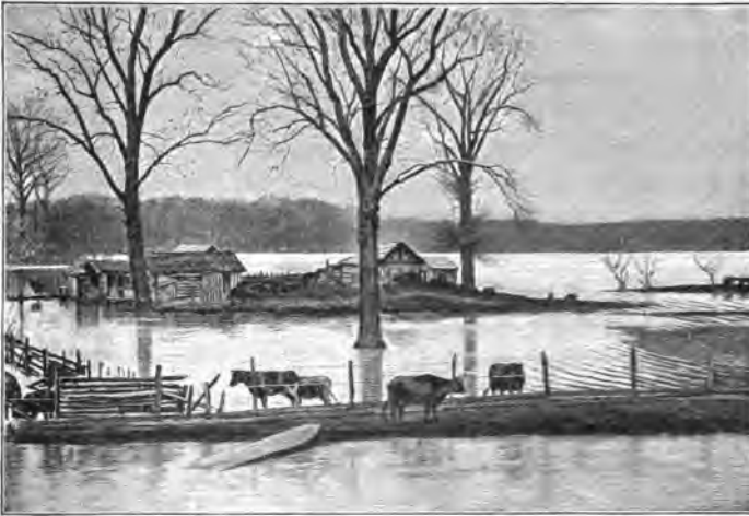
Flood Caused by a Break in a Levee.
